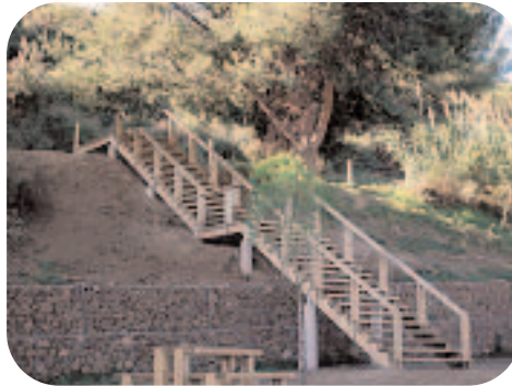
Creation of a stepped walkway after the rehabilitation operation
